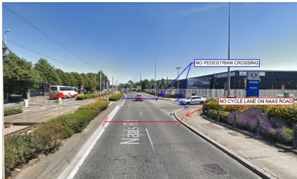
Figure 11.1.4 – Existing Naas Road Pedestrian/Cyclist Facilities
