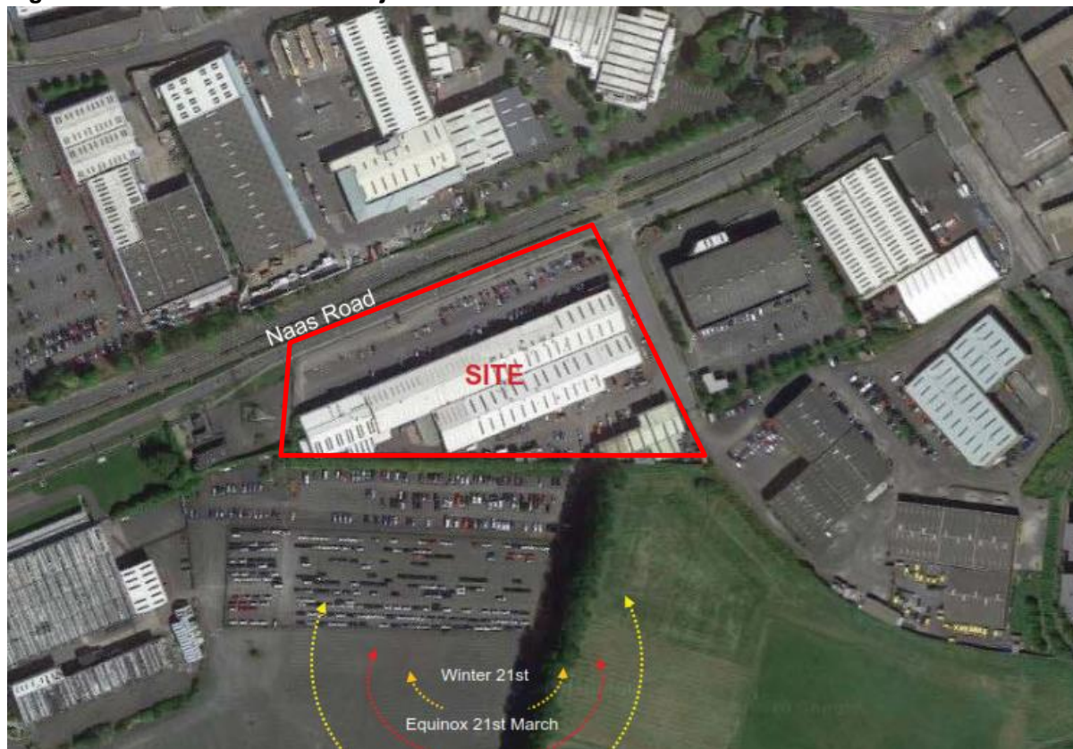
Figure 3.4: Aerial view of the subject site
